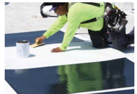
Clean & Prep TPO
