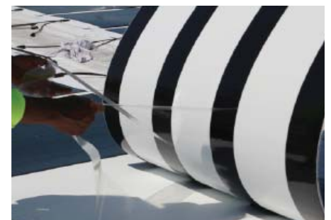
Peel & Stick Modules to TPO
