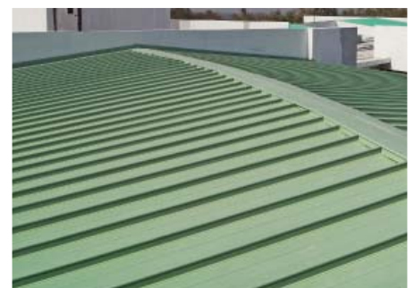
Steep-slope Standing Seam
