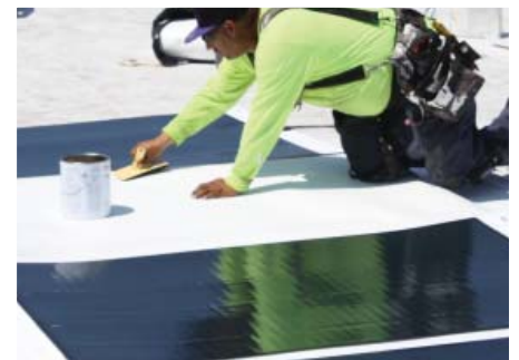
Clean & Prep TPO
