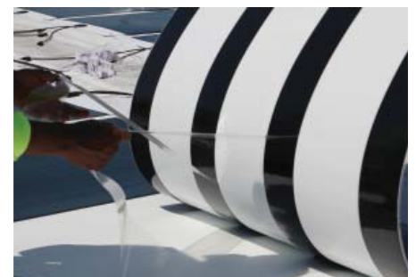
Peel & Stick Modules to TPO
