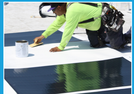
Clean & Prep Membrane Roof
