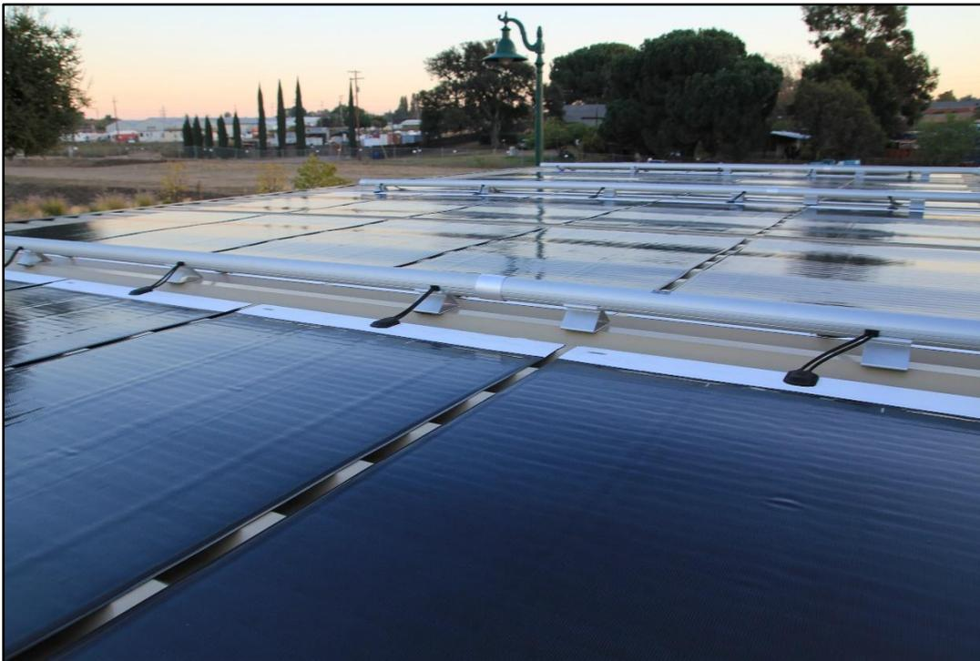
Figure 5 Completed Solar Carport with Wire Management
