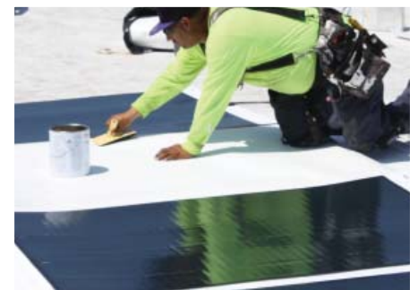
Clean & Prep TPO
