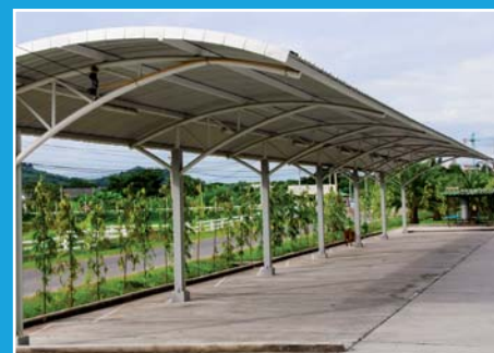
Solar Parking Canopies
