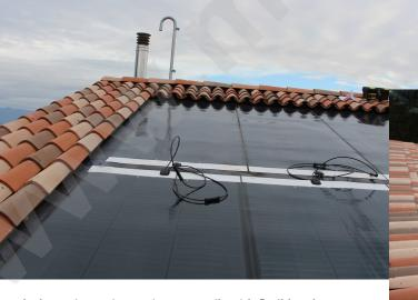
The house in Trevignano integrates tile with flexible solar, without the need for racking. From the street, the solar system is barely visible on the two story house.
